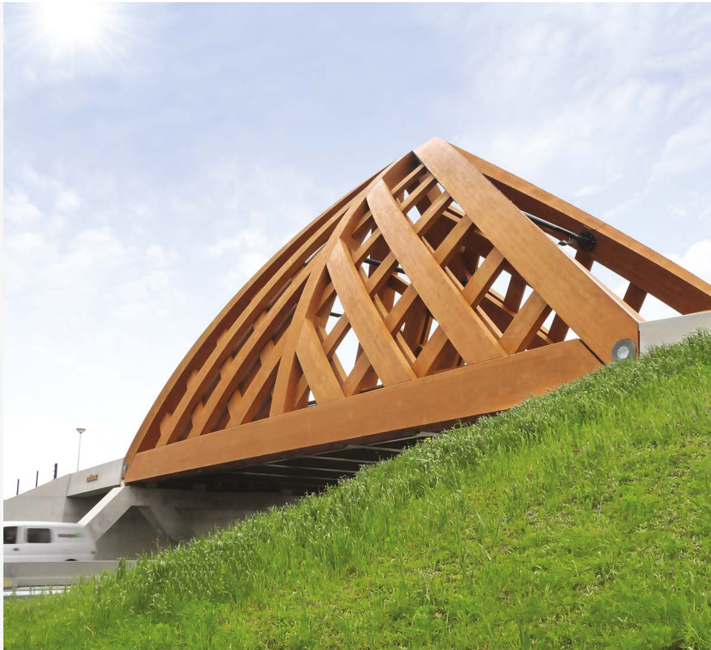
SNEEK BRIDGE THE NETHERLANDS
